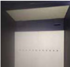
4. Place inner baffle on brackets
